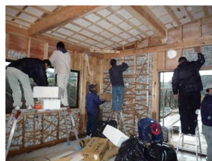
The members fill in old news paper into the wall for the insulation .
