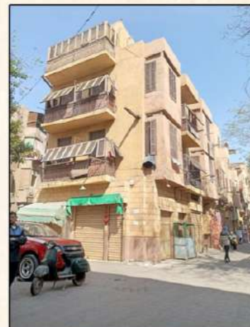
3d for houses after restoration
