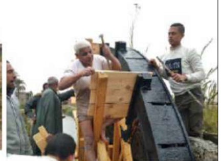
Image 28: Installing the waterwheel
