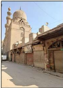
Rabbe Al manistrili before dilapidated 2022
