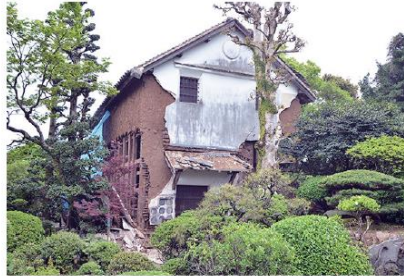
Photo 3.1.1.4 The central storehouse (after the earthquakes)
