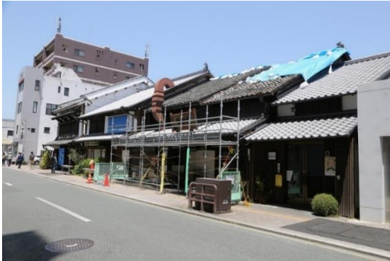
Damaged town houses
