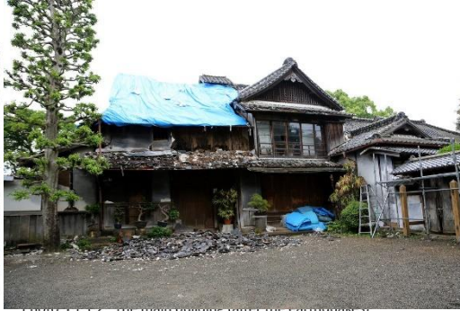
Photo 3.1.1.2 The main building (after the earthquakes)
