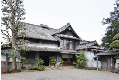
Photo 3.1.1.1 The main building (before the earthquakes)
