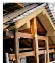
Repair of beams and columns of cultural property buildings
