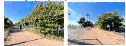
Current status of well overgrown trees after 10 years
