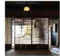
Replacement of shoji paper screens
