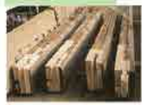
Repair of end joints of wooden parts such as columns and beams of cultural property buildings
