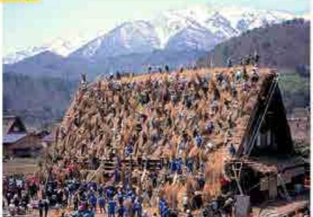
Rethatching at a thatched roof through "Yui" and volunteers.
